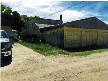
W/SW – 4-unit Apartment Building
