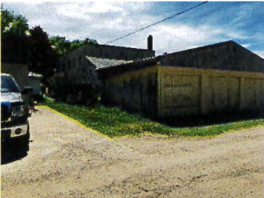
W/SW – 4-unit Apartment Building
